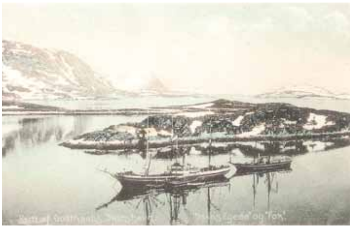
Figure 2. Two new steamships in the Godthaab harbour. "Hans Egede" being the first steel ship.
